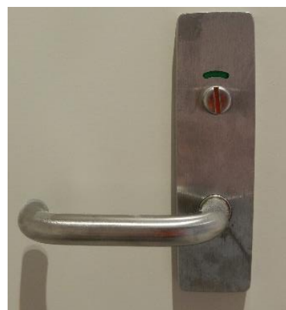
The above image indicates a privacy latch set provided to accessible WC facilities as viewed from the outside
