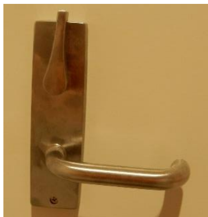
The above image indicates a privacy latch set provided to accessible WC facilities as viewed from within the facility
